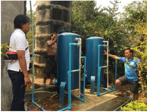
Villagers in Huai Ya No, one of the sub-villages of Huai Kang Pla, installed water filtration tanks. © IUCN/Angela Jöhl Cadena
