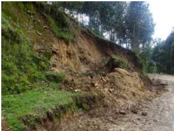
Figure 15: Road embankment failure on feeder roads in Sebeya catchment.
