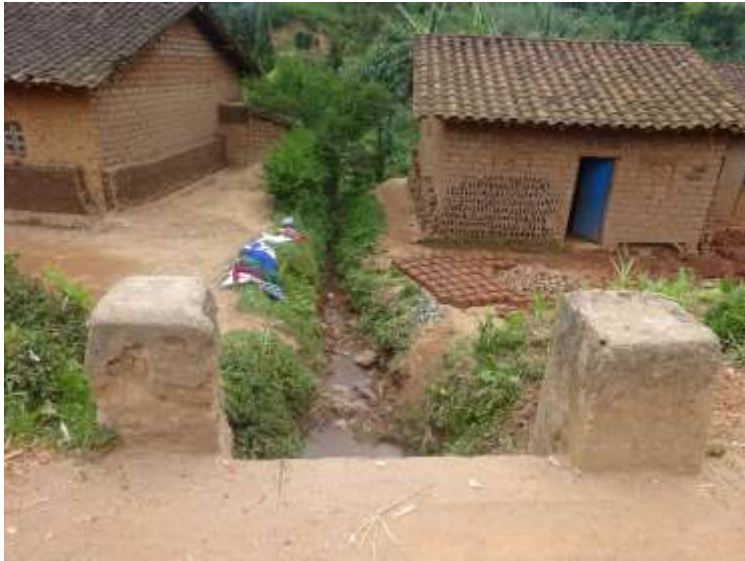
Figure 14: Road runoff crosses roadway posing risks to communities' buildings.
