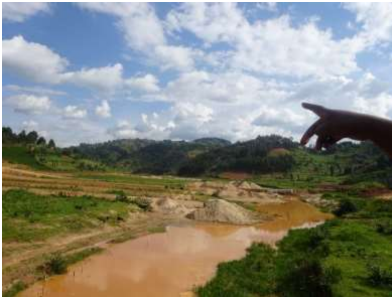
Figure 19: Dam under construction Sebeya catchment.
