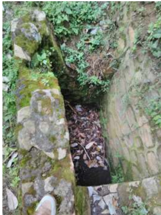
Figure 13: Culverts partially and fully clogged on feeder roads in Sebeya catchment.
