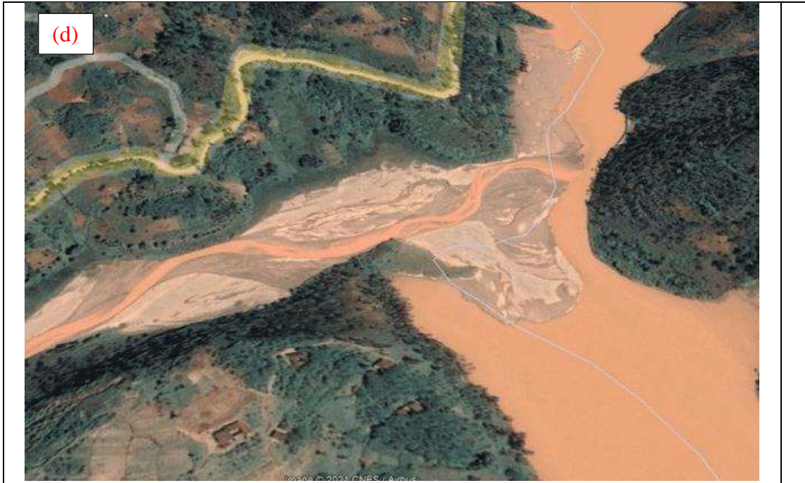
December 2020: huge quantity of sediment deposited in NyabarongoI hydropower
