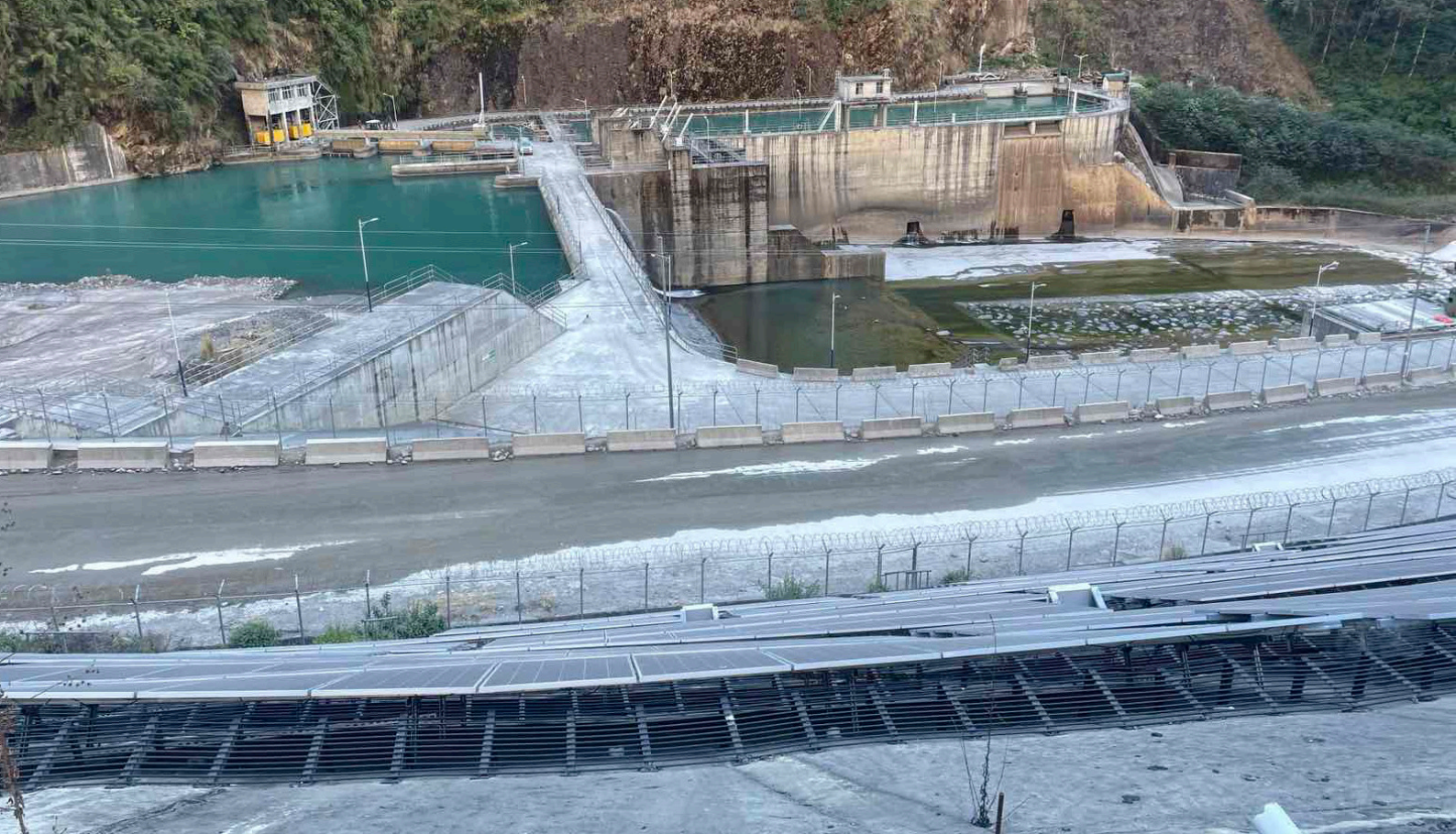
Reservoir of Upper Bhotekoshi hydropower plant in Sindhupalchowk, Nepal.
