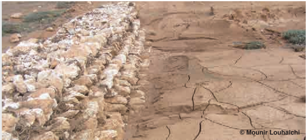
Figure 2. Stone wall to control water erosion in the landscape
