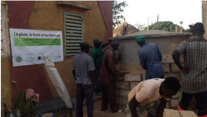
Photo: Rainwater Harvesting Tank construction. Florian Biesle, IRHA.
