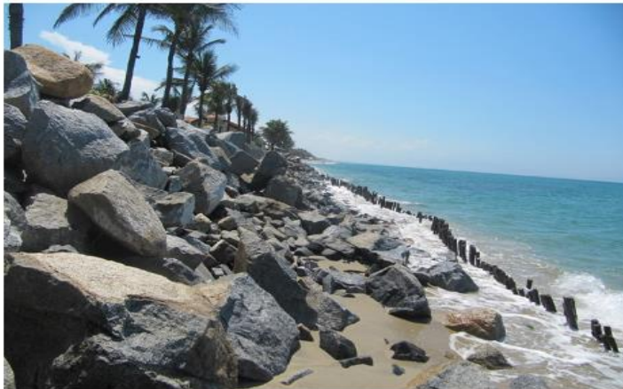
Rocks on the Cửa Đại beach have been used to protect a local resort.
